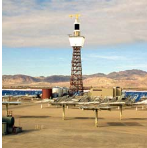
Solar Two in Nevada uses molten salts as storage for solar energy.
