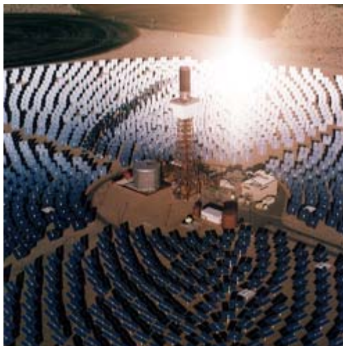
Solar panels in Nevada
